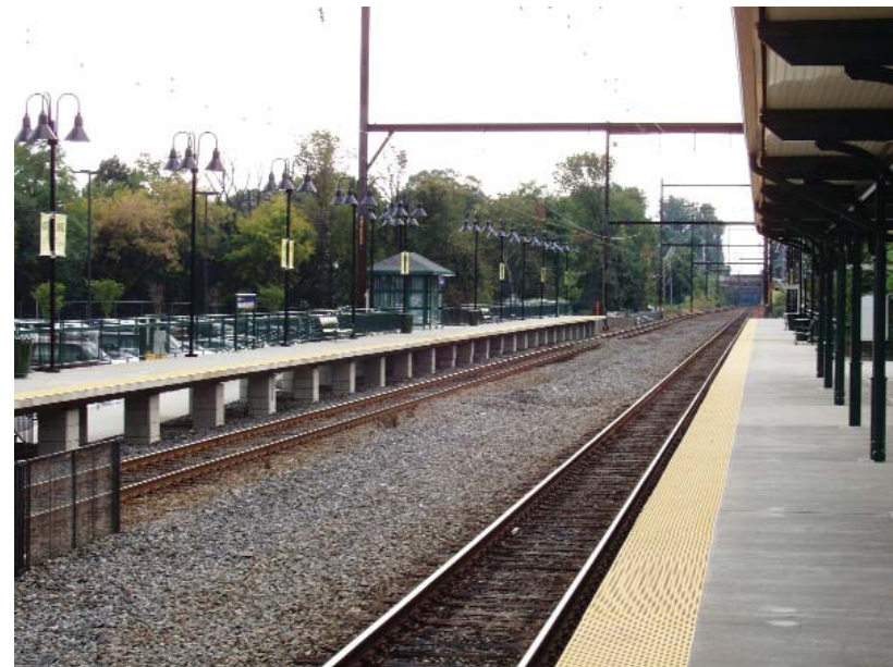
View of high level platform.
