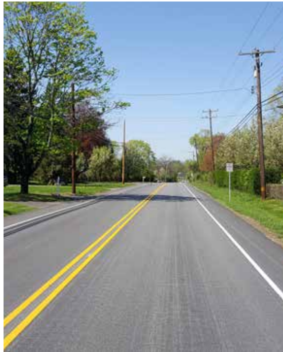
Tar and chip paving is an effective solution for rural roads, but the loose gravel it creates makes it tough to bicycle on.
