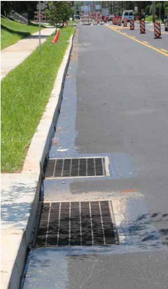
Bicycle-safe drainage grates typically have a matrix pattern that prevents tires from becoming stuck in them, like this one installed along Markley Street in Norristown.
