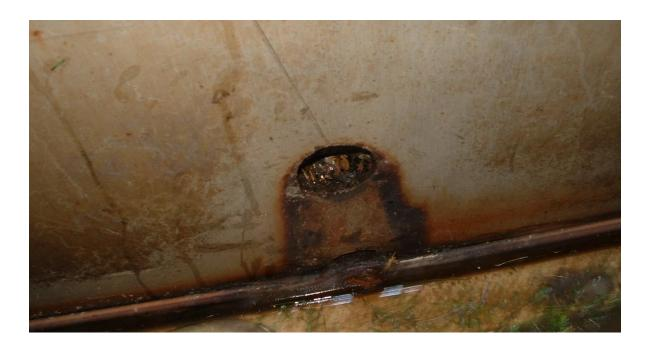
A two-inch diameter hole is cut in the bottom third of the stainless steel sheet that meters the water from the one side of the manhole to an outlet on the other side of the manhole. The outlet runs underground to a manhole that is connected to the existing storm water piping network at the end of Fairway Drive.
