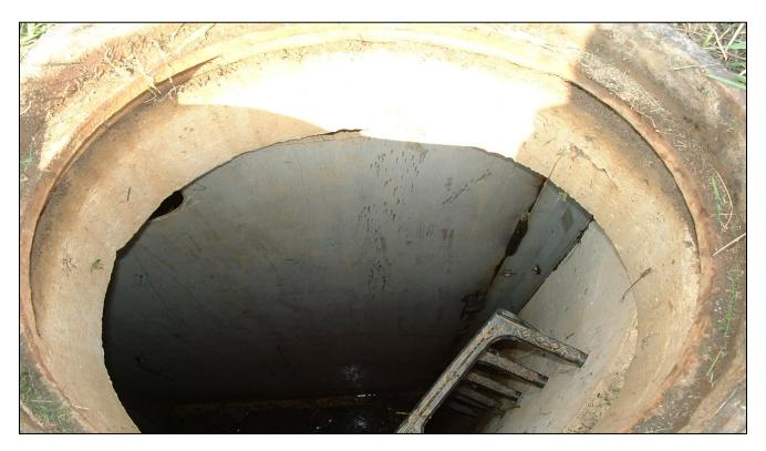
The manhole contains a five-foot by 10-foot sheet of stainless steel that bisects the manhole and acts as a baffle.
